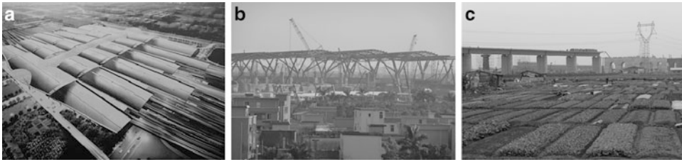
Fig. 4.4 Conceptual design of the Guangzhou South Railway Station (a) and construction sites of the railway station project in Shibi Village in 2009 (b and c) (Strohschön et al. 2013)
