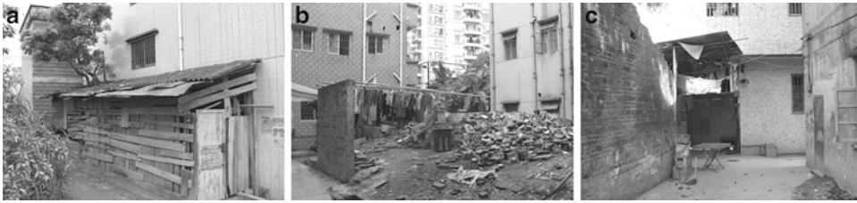
Fig. 4.7 Temporary constructions: solitaires or additional space on/at existing building (a), unused areas as storage surfaces and floor spaces (b), and composition areas for
