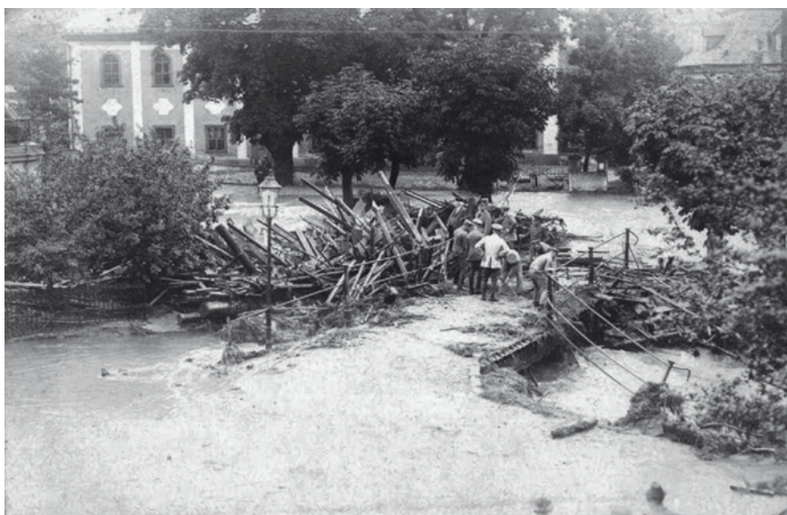
Fig. 18.4 Jelenia Góra-Sobieszów (PL): Woody depositions on the bridge after the flood 1897 blocked stream channel in the Bóbr/Bober R. basin ( http://wroclaw.hydral.com.pl )
