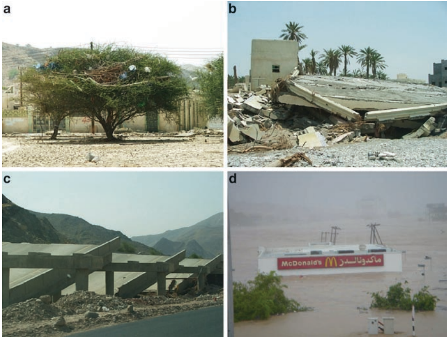
Fig. 4 Wadi runoff: (a) high water marks in the form of rafted debris in a tree at Hail al Ghaf located 7 km inland and at 50 m elevation; (b) pancake collapse of a building due to foundation scour at Quriat (c) highway bridge collapse due to uplift forces in the mountains south of Muscat; (d) Wadi flooding due to discharge and storm-surge-induced backwater at Muscat (Photo credit: Department of Meteorology, Sultanate of Oman)
