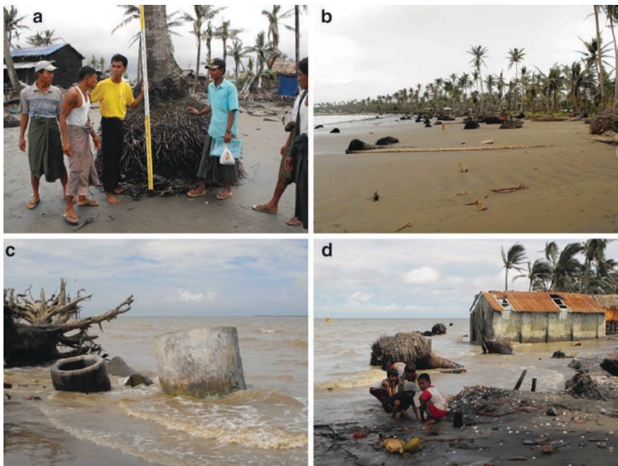
Fig. 4 Coastal erosion: (a) survey of vertical erosion on palm tree roots at Aung Hlaing; (b) beach erosion at Kyauk Ka Latt; (c) drinking water wells scoured in surf zone at Aya; (d) Golden Buddhist Stupa built on land piercing the water surface offshore highlighting 150 m land loss
