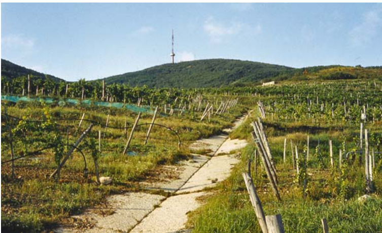
Plate 7.6 A concrete road also functioning as a drainage ditch between terraced irrigated vineyard plots, in the vicinity of Tarcál (Tokaj-Hegyalja Region) (Csorba 1985)
