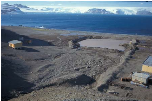
Plate 16.1 Storage basin between dykes near the buildings of the Arctowski Station on Antarctica (Nagy 2003)
