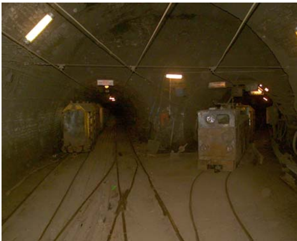
Plate 10.2 A shaft section of the main pit in Lyukóánya secured by a concrete frame and steel rings (Sütő 2003)
