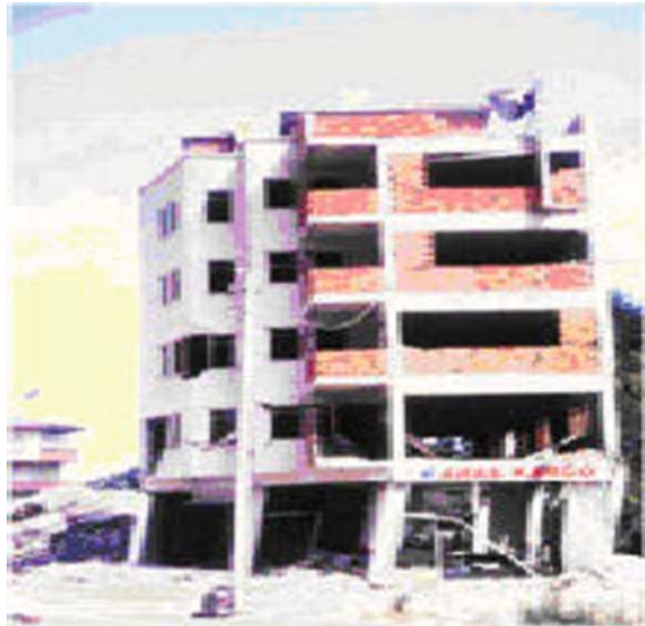
Fig. 16.2 Side sway mechanism with incipient collapse (See also Plate 20 in Color Plate Section on page 467)
