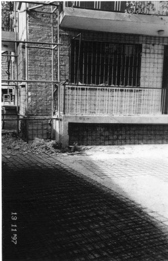
Fig. 8.23 Application of web reinforcement
