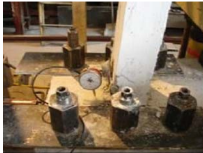
Crushing of cover concrete
