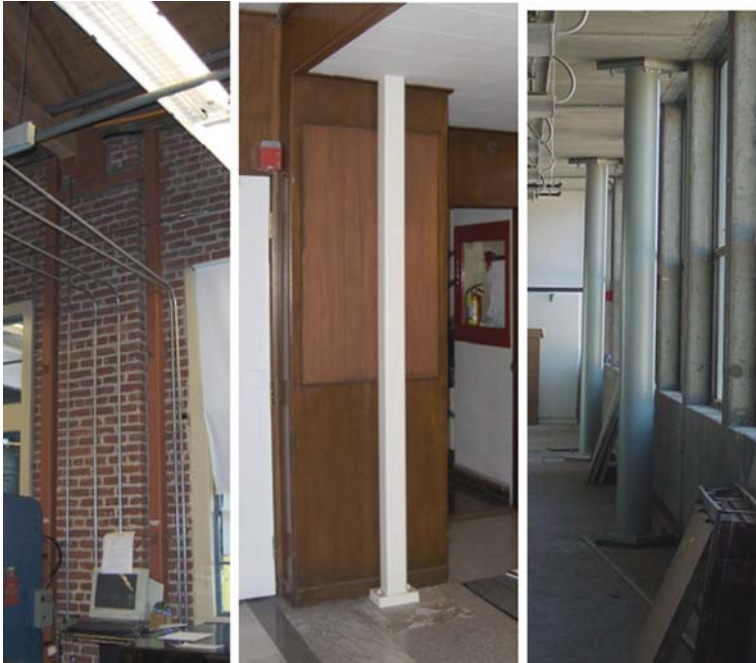
Plate 21 Steel column “pre-shoring” examples from Stanford University and University of California, Berkeley (see also Fig. 16.3 on page 331)
