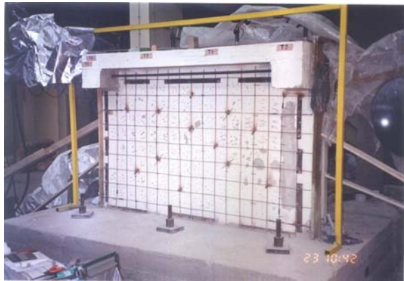
Fig. 19.13 Integrated wall and strengthening by wire mesh (See also Plate 32 in Color Plate Section on page 473)
