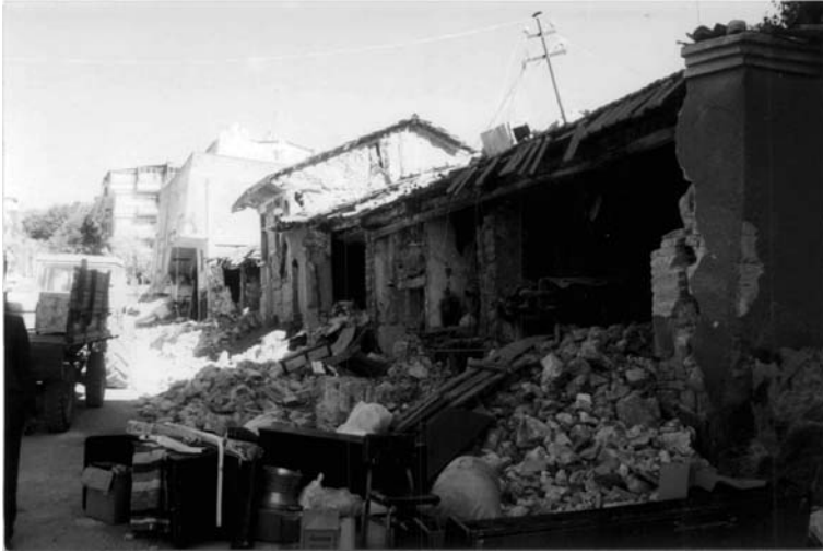
Fig. 8.6 Substandard wall units
