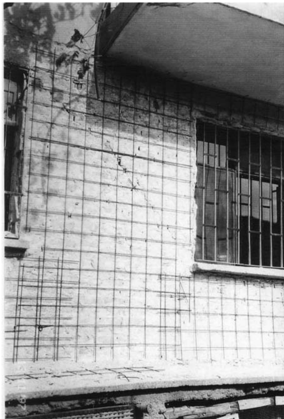
Fig. 8.24 Application of web reinforcement
