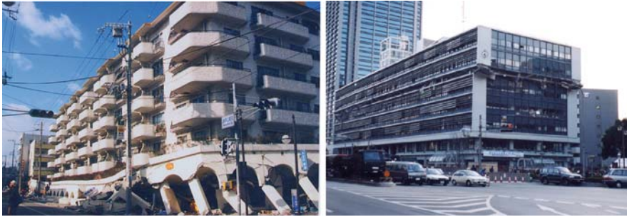
Fig. 11.1 Damages of soft-first-story buildings during Kobe earthquake (See also Plate 14 in Color Plate Section on page 463)
