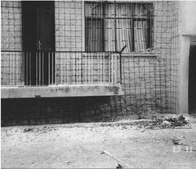
Fig. 8.25 Application of web reinforcement
