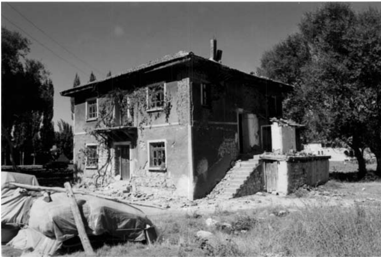
Fig. 8.7 Substandard plaster
