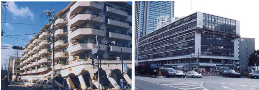
Plate 14 Damages of soft-first-story buildings during Kobe earthquake (see also Fig. 11.1 on page 212)
