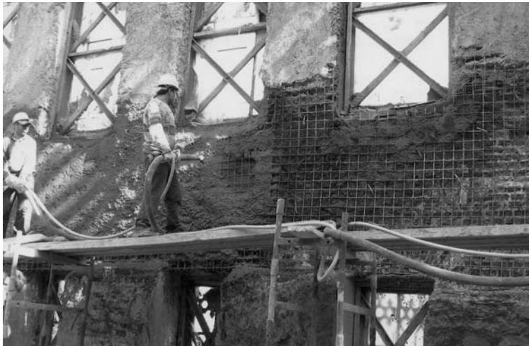
Fig. 8.26 Application of shotcrete
