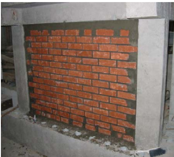
Fig. 19.16 Strengthening of a bare frame by integrated high strength bricks (See also Plate 35 in Color Plate Section on page 474)
