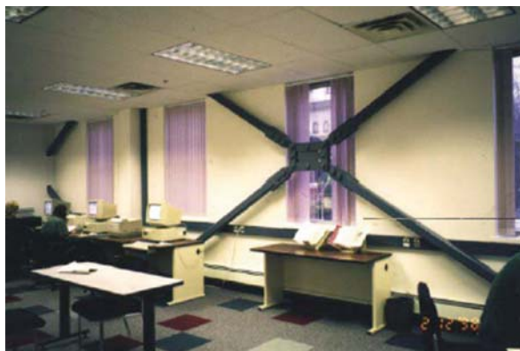
Fig. 6.12 X-braced friction damper in Harry Stevens Building
