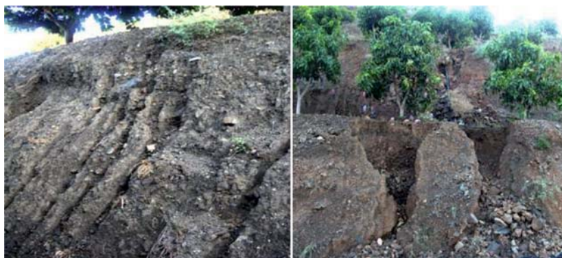
Fig. 7 Rills and gullies in the taluses of orchard terraces
