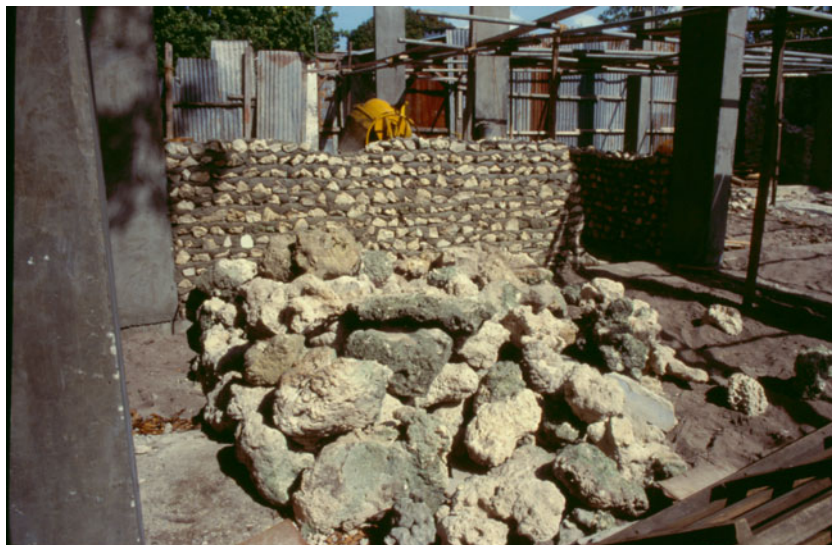
Mining/Quarrying of Coral Reefs, Figure 1 Example of the use of coral rock in construction in the Maldives.
