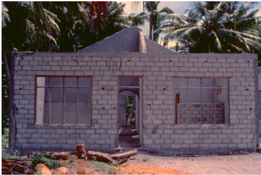
Mining/Quarrying of Coral Reefs, Figure 4 The use of concrete blocks in construction in the Maldives.
