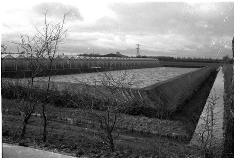
Picture 6.2 A basin for storage of rain water
