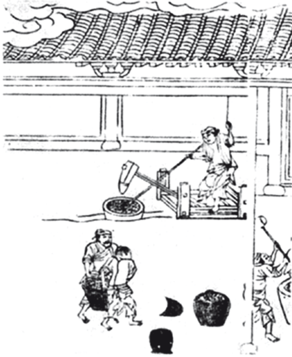
Fig. 2.10 Foot-operated hammer (From the Kêng Chih Thu [86])
