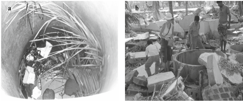
Fig. 1 Tsunami impact on open well and the general devastation of the coastal area in east Sri Lanka ( Courtesy a: Scott Tylor and Jayantha Obeysekera; b: Karen Villhloth ).
