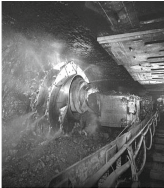
Fig. 8 New automation technology designed to locate and guide coal-cutting equipment in longwall mines (Hill-Douglas, 2007).
