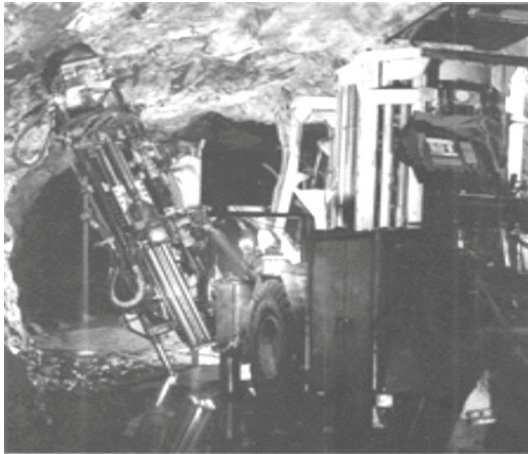
Fig. 19 A load-haul-dump vehicle in LKAB's iron ore mine in Sweden scoops rock with the help of a teleoperator working off-site; the vehicle does hauling and dumping automatically (DeGaspari, 2003).
