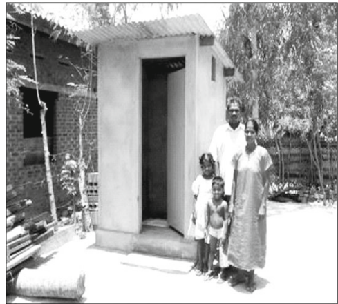
Fig. 4 Typical permanent toilets built for a private housing for a 4-rescue family.
