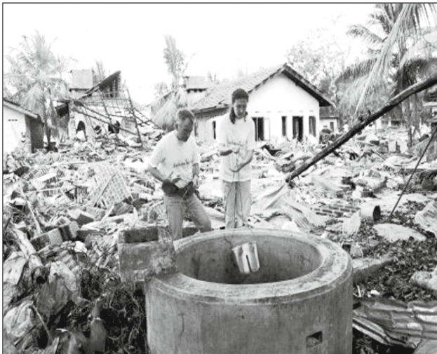
Fig. 5 Typical water well in the area: accessibility for water analysis was difficult due to the large amount of solid wastes surrounding the well.
