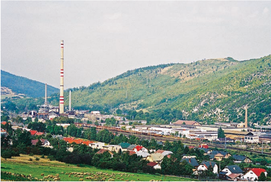
Plate 27 Copper smelter at Krompachy, Slovakia (2002). Note development of industrial barren and extensive soil erosion on the hill behind the smelter. Photo: V. Zverev
