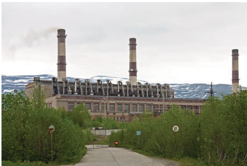
Plate 1 Power plant at Apatity, Russia (2008). Photo: V. Zverev
