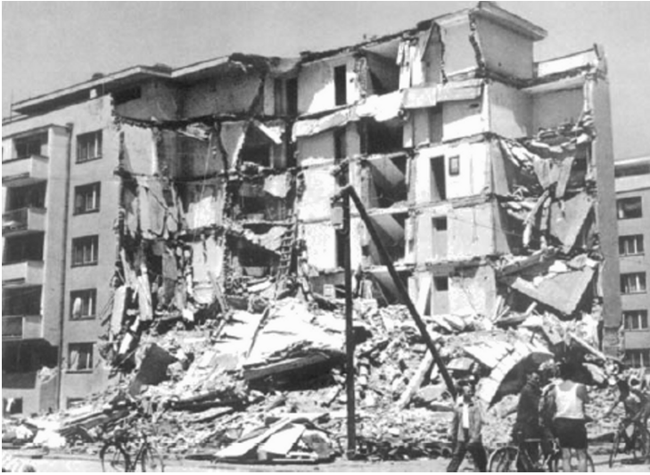
Figure 4. Total collapse of URM building, Skopje 1963 (Petrovski, 2004)
