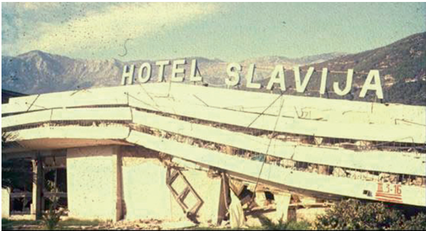
Figure 8. Soft-story and non-symmetrical structure Montenegro 1979
