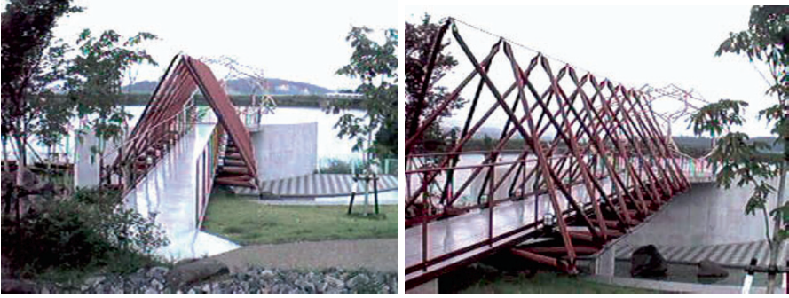
Figure 28. Deployable bridge in Hamanizuki Park
