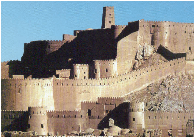
Figure 12. The old city of Bam in south-east Iran before the earthquake
