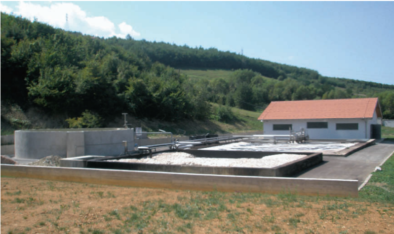
Figure 13. Membrane – biological reactor (MBR) at the Sarajevo sanitary landfill (Serdarevic, 2008)
