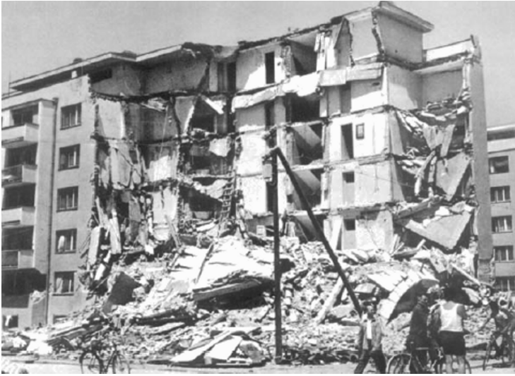
Figure 4. Total collapse of URM building, Skopje 1963 (Petrovski, 2004)
