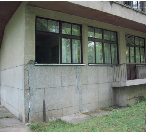
Figure 7. Measured settlements was 28 cm
