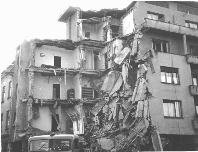
Figure 5. Partial failure of the masonry building, Banja Luka 1969
