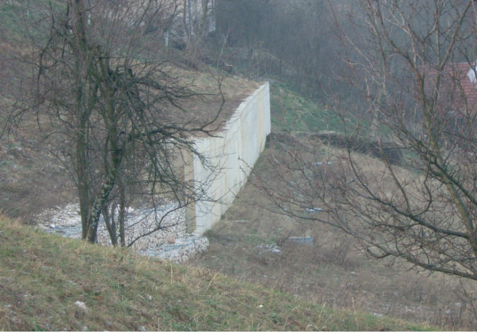
Figure 19. Finished retaining structure
