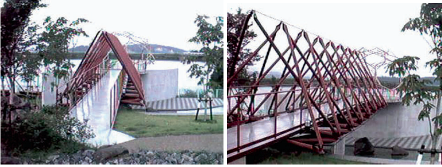
Figure 28. Deployable bridge in Hamanizuki Park
