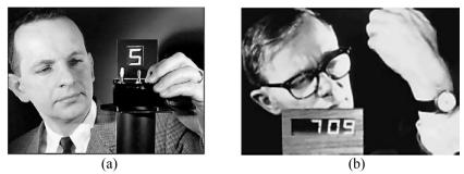
Fig. 2.4 RCA prototypes. (a) Heilmeier shows one of the first LCDs based on dynamic scattering. (b) The first LCD digital clock
