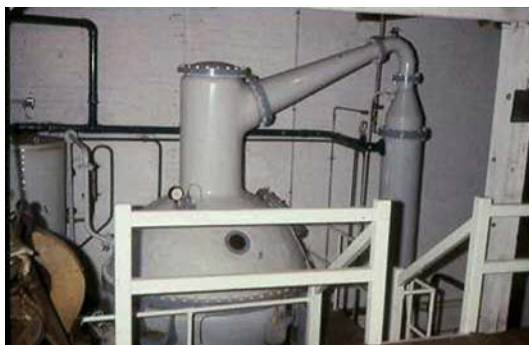
Figure 8.9 Vinegar distillation plant
