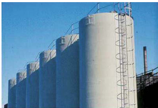
Figure 8.6 Storage tanks of malt vinegar after acetification
