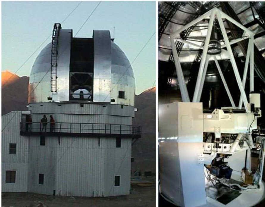
Fig. 6.11 Left: The 2 m HCT dome, with the telescope seen through the dome slit. Right: A closer, full view of the telescope inside the dome
