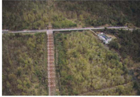
Fig. 5.27 An aerial view of the Mauritius Radio Telescope, as seen from the south. A part of the east-west arm with fixed helices is visible in the upper part of the figure. Sixteen trolleys with four helices each are seen in the south arm.
