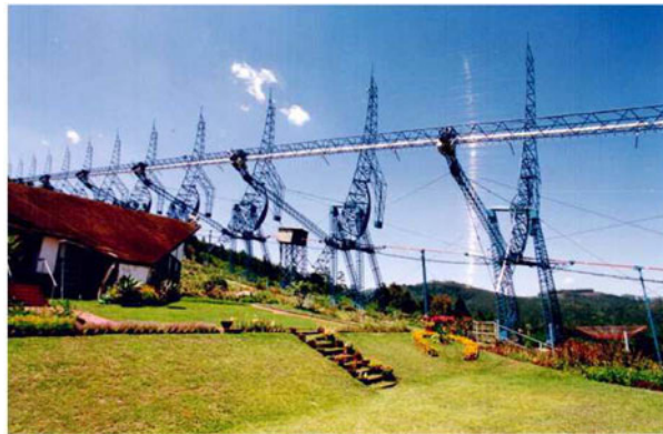
Fig. 5.3 ORT consists of a 530 m long and 30 m wide parabolic cylinder with its long axis parallel to that of the earth; the long white streak on right side is reflection of 1,100 stainless steel wires by the sunlight (Swarup et al. 1971)
