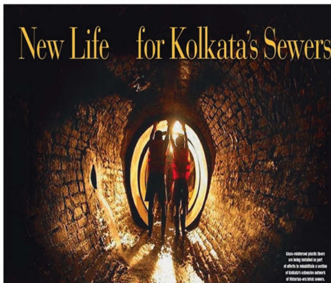
Fig. 13.12 A completed section of lined brick sewer
