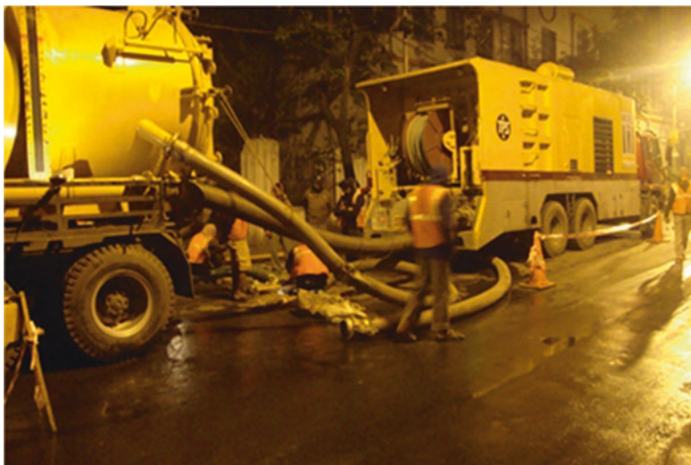
Fig. 13.8 Super sucker used for desilting of sewers at night
