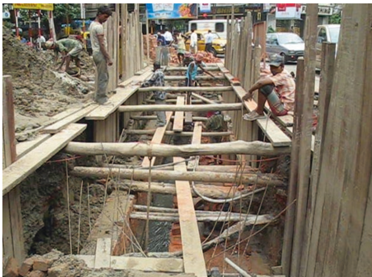
Fig. 13.7 A typical sewer repair by conventional open cut and cover method
