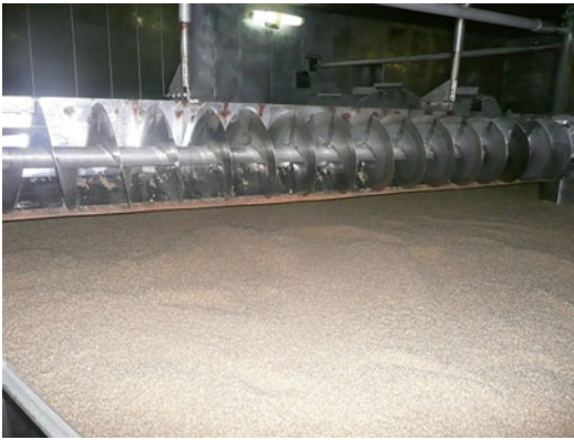
Fig. 9.5 Automatically controlled koji making machine
