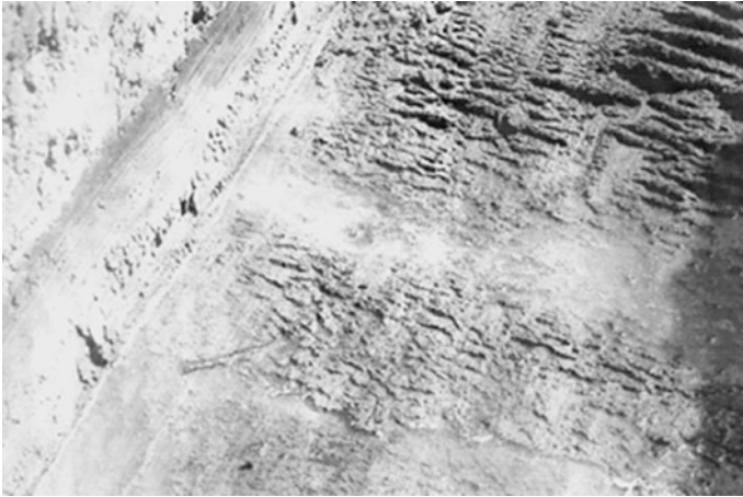
Fig. 21.11 The early aspect of pipe forming through the sandy silt under excessive gradient. Picture taken 4 min after picture of Fig. 21.10
