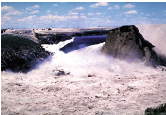
Photo 10.1 Teton Dam, Idaho, June 5, 1976 from http://en.wikipedia.org/wiki/Teton_Dam
