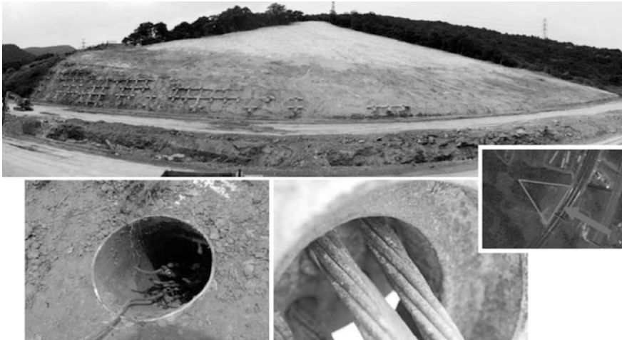
Fig. 15.5 Failure plane of the studied slope (Lee et al. 2013)
