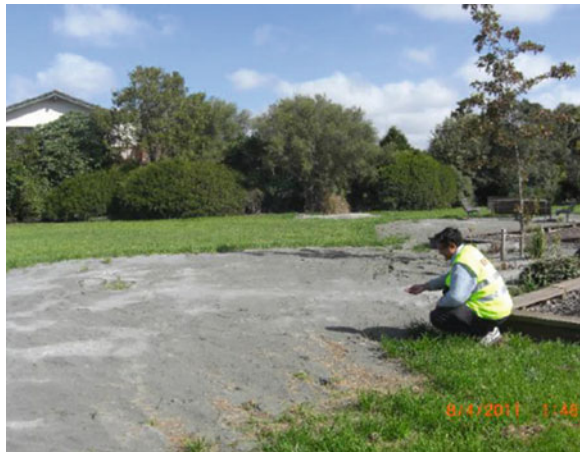
Fig. 28.2 Sand boils due to soil liquefaction
