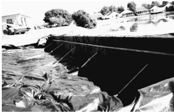
Fig. 33.13 Close-up of geotextile lay down and wrap up on timber bulkhead
