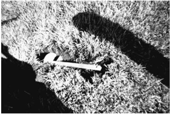
Fig. 33.10 Setting up of the tie back helical anchor
