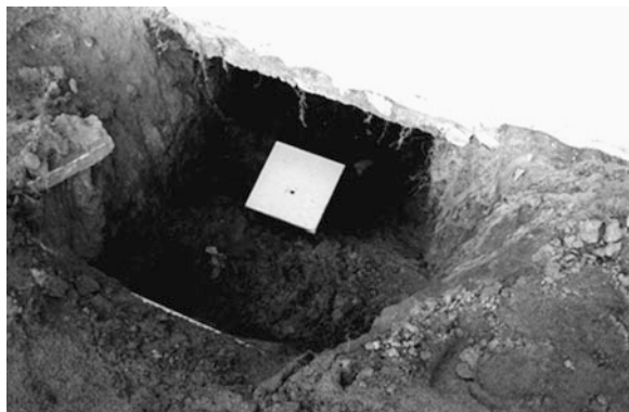
Fig. 33.8 View of helical support anchor in place
