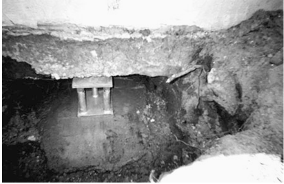
Fig. 33.9 View of support cap and bracket assembly under the footing
