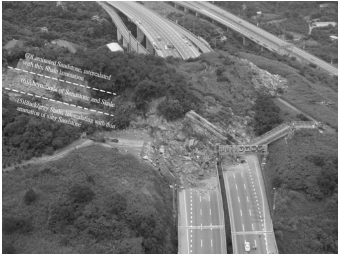
Fig. 15.10 Aerial photo of dip slope failure (Lee et al. 2013)
