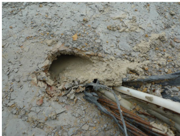
Fig. 15.7 Unsealed free anchor end found from anchor remained on sliding surface
