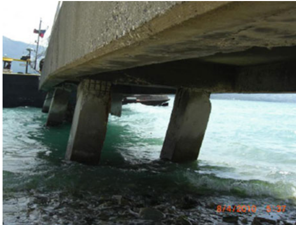
Fig. 28.14 Hinging of piles supporting a wharf structure
