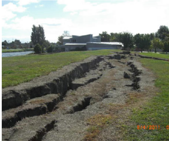
Fig. 28.4 Lateral spreading following soil liquefaction
