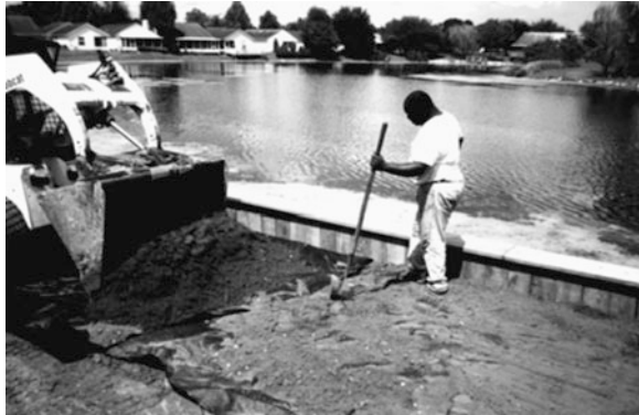
Fig. 33.15 Additional fill being dozed into the anchored geotextile
