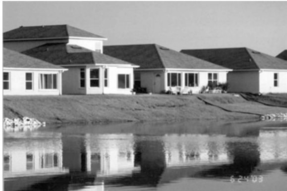
Fig. 33.1 Close-up view of the subsided backyard
