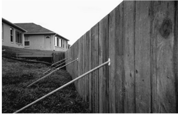
Fig. 33.12 Close-up the helical anchor tie back with timber bulkhead
