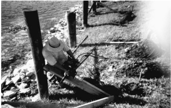
Fig. 33.11 Hydraulic setup for achieving torque/resistance capacity
