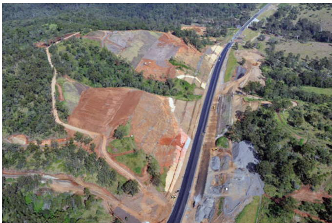
Photo 16.4 Cut 3 south and Cut 4 south, after crest removal March to June 2009
