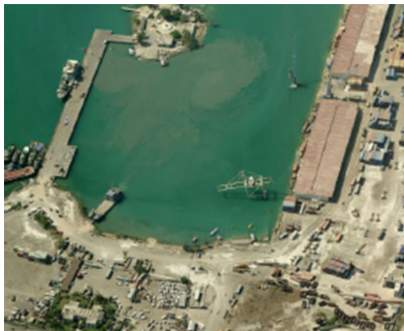
Fig. 28.12 Pictometric image showing the damaged crane structure
