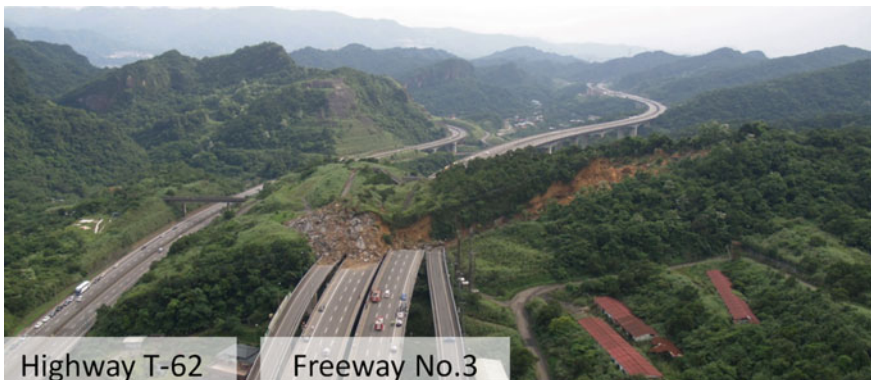
Fig. 15.1 Freeway No. 3 Landslide (after Liao and Lee 2011)
