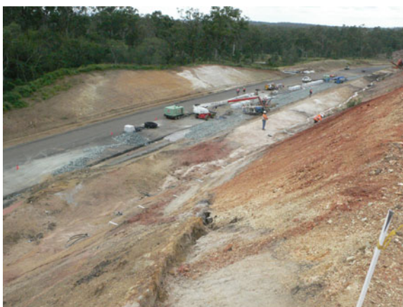
Photo 16.3 Movement along contact zone, Bench 2 to Bench 3, Cut 3 south. February 2008
