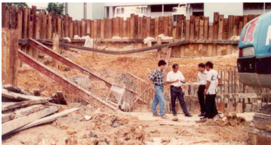
Fig. 18.2 Problem of diagonal corner steel strut
