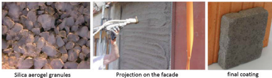
Fig. 10 The new aerogel-based insulating coating ( rendering )
