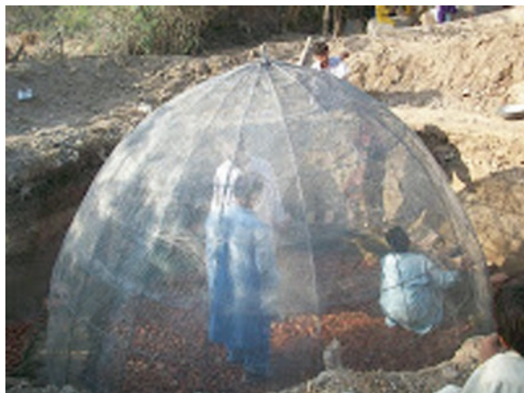
Fig. 11 Ferro-cement biogas plants (Construction of a biogas plant in Mirpurkhas Sindh Pakistan 2012)
