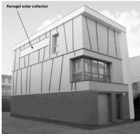
Fig. 7 Solar thermal collector with aerogel glazing integrated to building facade (Dowson et al. 2012)
