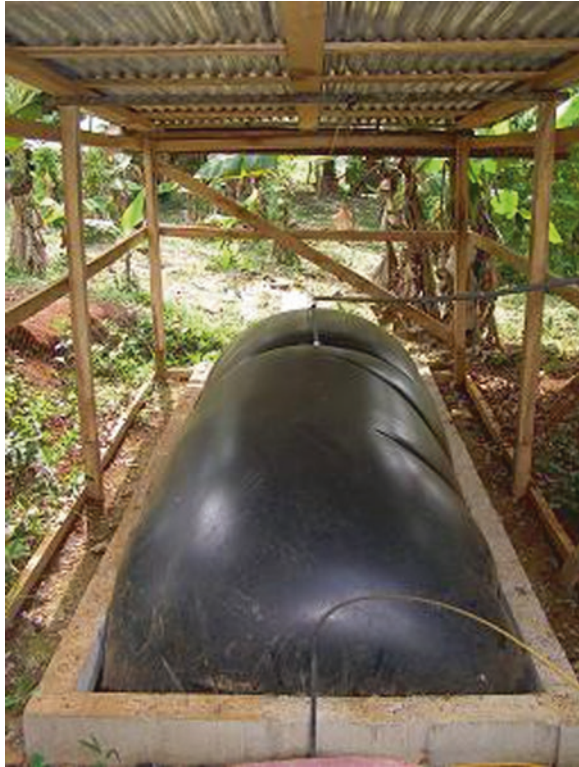
Fig. 7 Balloon digester as seen in Costa Rica (see footnote 16)
