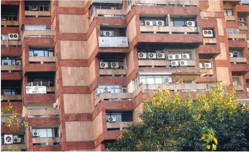
Fig. 3 Picture showing multiple electrical air conditioners installed at a typical building
