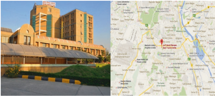
Fig. 5 Demonstration site JPNATC, AIIMS in New Delhi
