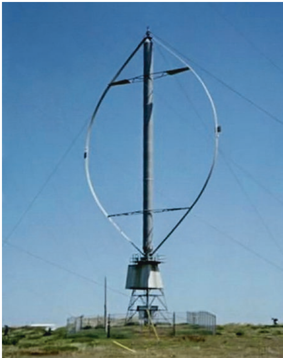
Fig. 4 Darrieus wind turbine. Source http://en.wikipedia.org/wiki/Darrieus_wind_turbine
