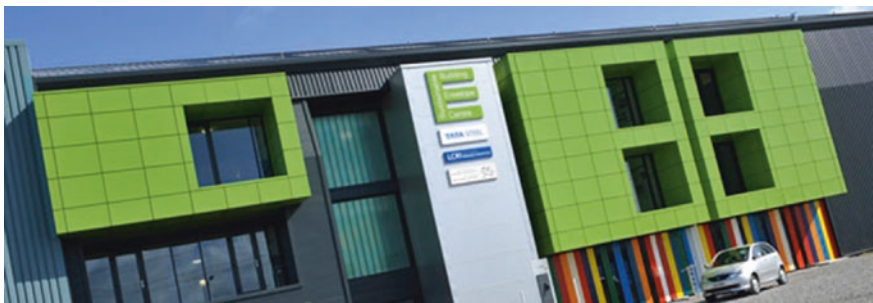
Fig. 11 Sustainable building envelope centre, Shotton, Tata Steel, Deeside, United Kingdom
