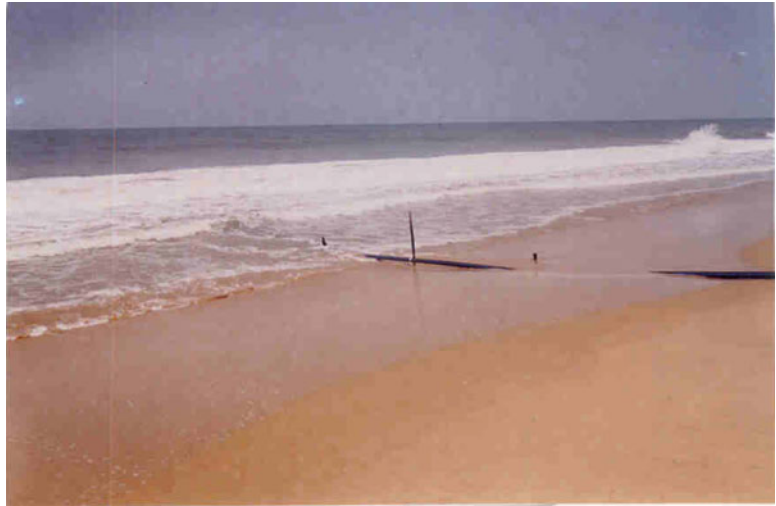
Plate 4 Seawater intake system
