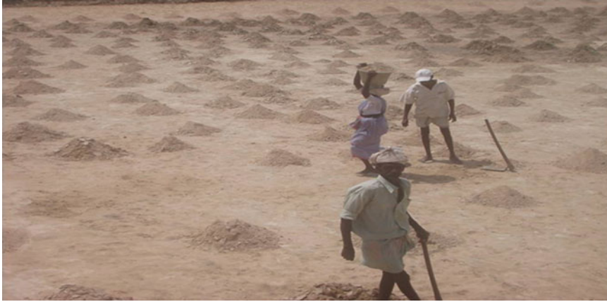
Scraping the pond bottom (using man power)
