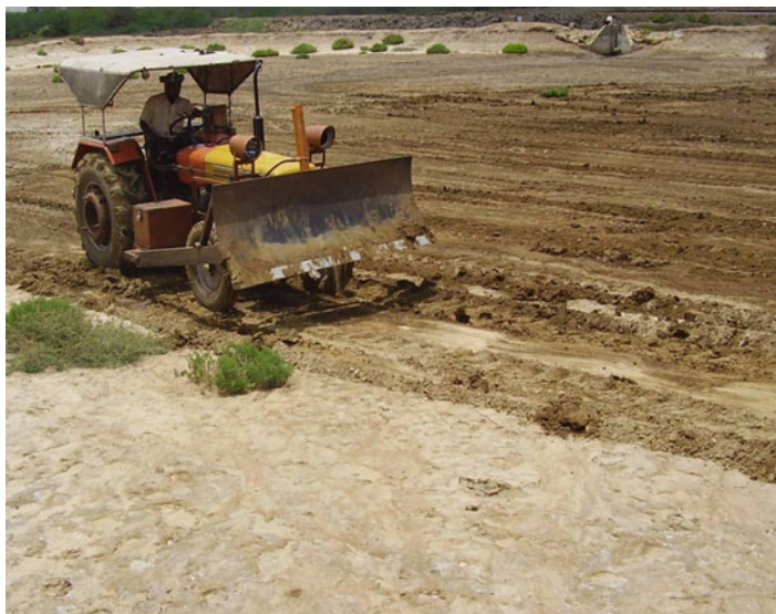
Renovating the pond (using tractor dozer)
