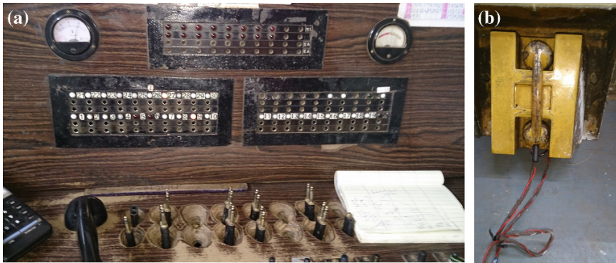
Fig. 3 Communication system at site C. a Chord based communication board at surface. b Telephone set
