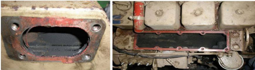
Fig. 6 Trap of soot at air cooler of the engine
