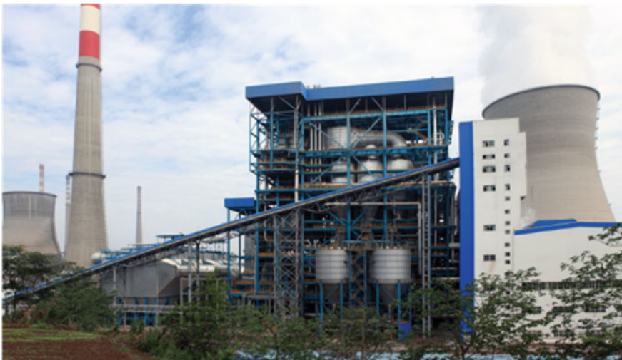
Fig. 2 The 600 MWe CFBC in Baima, Neijiang City, China, with supercritical steam cycle (Yang 2013)
