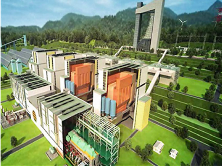
Fig. 3 The Samcheok project, 4 \times 550 MWe gross CFBs Korea (KOSPO 2016) with supercritical steam cycle
