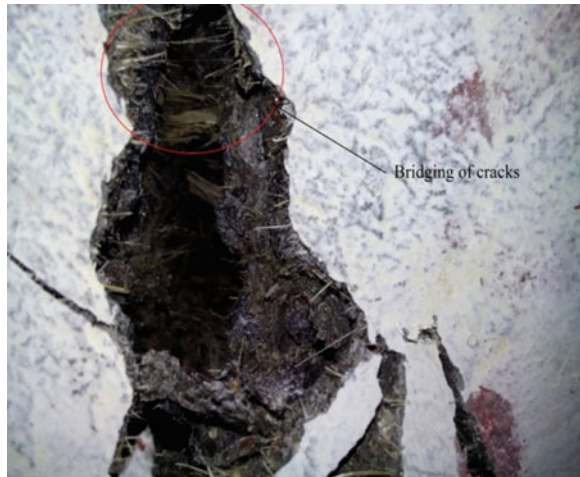
Fig. 14 Cylinder specimen of BFRC showing bridging of cracks by fibre
