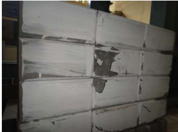
Fig. 5 Crack pattern due to out-of-plane load
