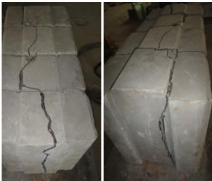
Fig. 12 Failure patterns when loaded parallel to the bed joint
