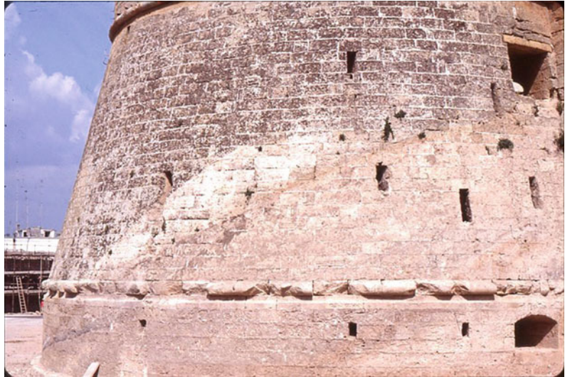
Fig. 9.14 Castle walls of Otranto, Italy—the area devoid of lichens demarcating the size and nature of a former earth embankment
