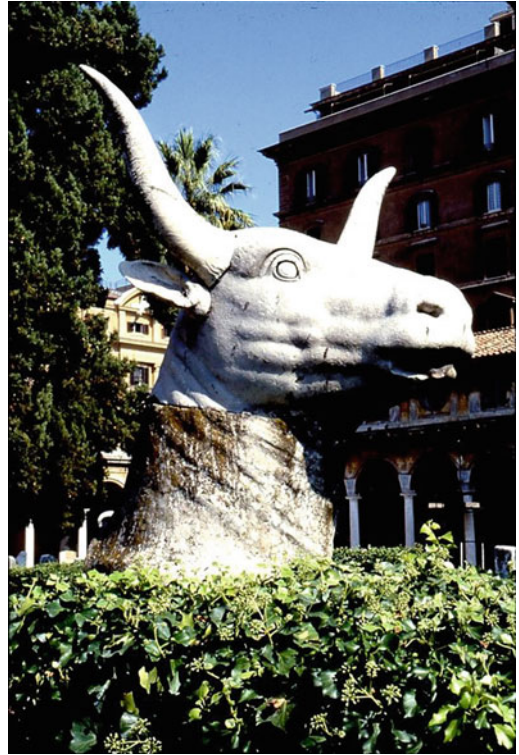
Fig. 9.13 Bull's head monument, National Museum, Rome—the use of non-authentic material (cement) for the neck providing a locus for non-characteristic and unappealing lichens to spread onto the marble sculpture
