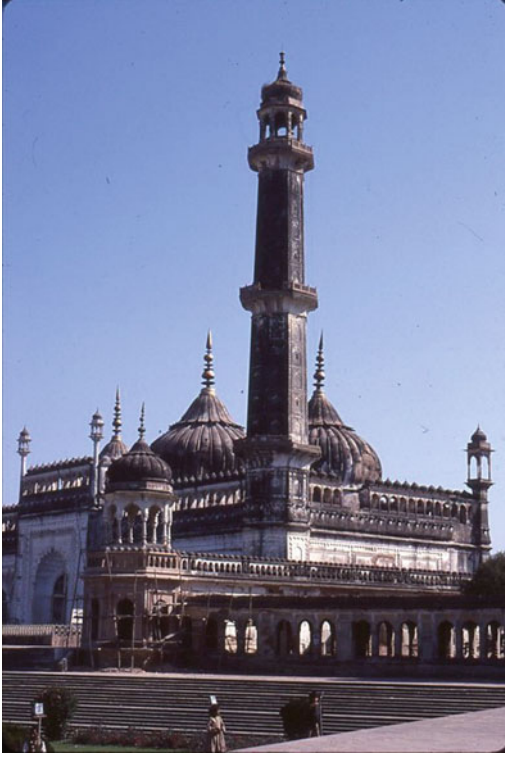
Fig. 9.7 Imam Bara Mosque, Lucknow, India—aesthetic disfiguration of building in a subtropical area, the dark biofilms created by both lichens and cyanobacteria
