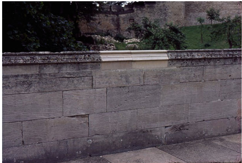
Fig. 9.10 Lincoln Castle, England—the restoration of a wall demonstrating the need for remedial action through the promotion of a suitable lichen assemblage
