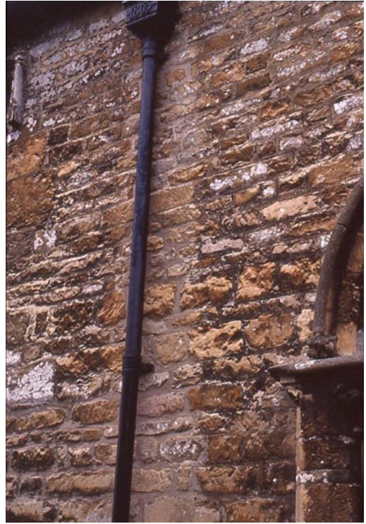
Fig. 9.9 Church wall, Fiskerton, England—the absence of lichen assemblages to either side of a metal downpipe clearly demonstrated
