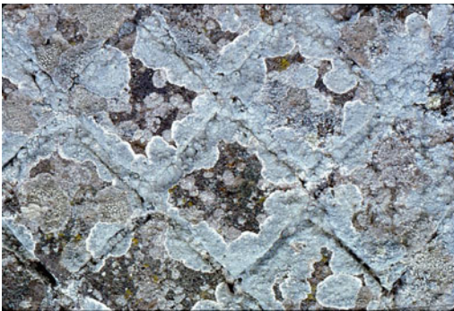
Fig. 9.12 Ostia Antica, Italy—the mortared areas of a characteristically reticulated Roman wall clearly generating a distinctive lichen assemblage
