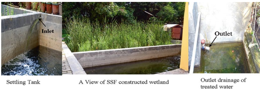
Fig. 3 Sub-surface flow constructed wetland at Shantikunj, Haridwar
