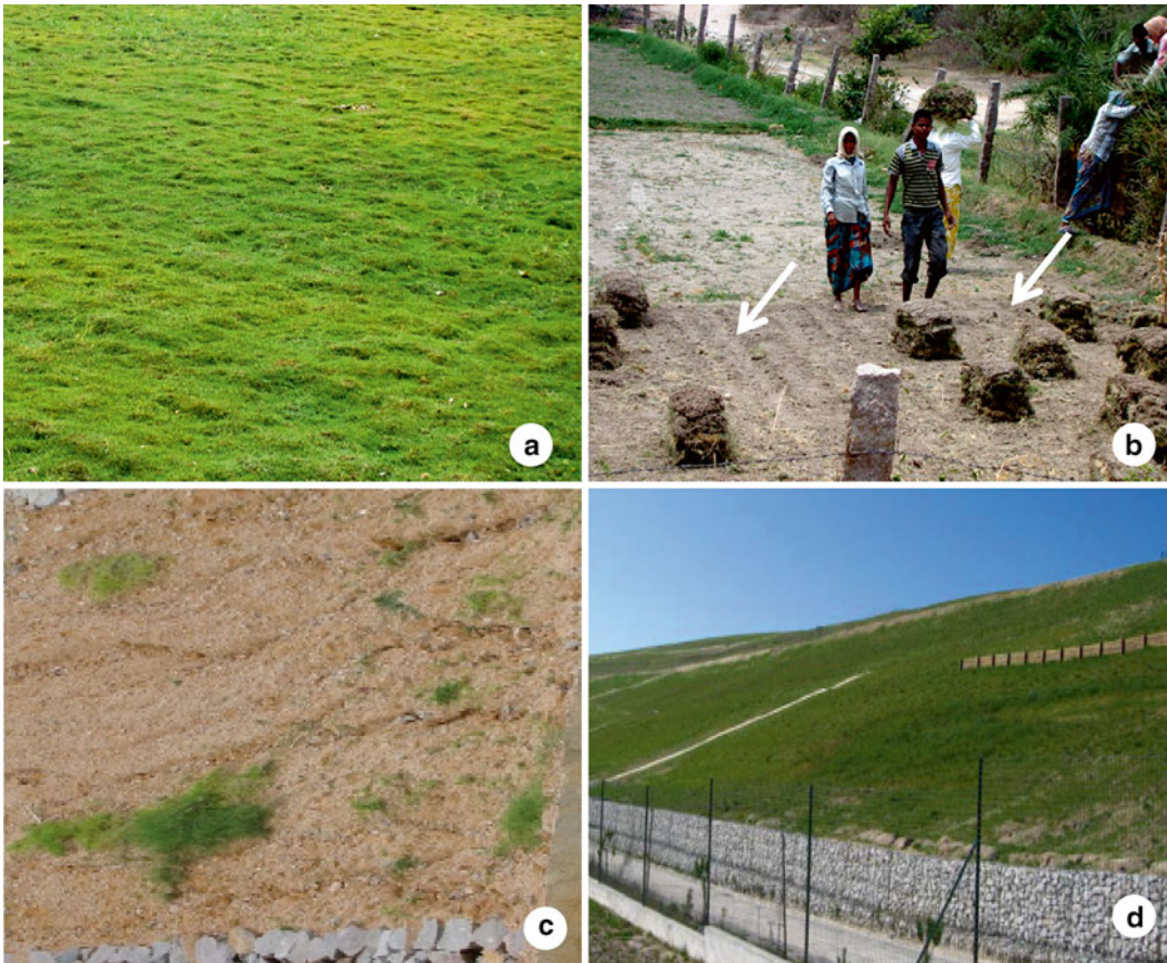
Fig. 5 Sodding, a bioengineering technique that uses grass mats for soil stabilization and erosion control. Perennial grasses are preferred. Grasses with sturdy adventitious root mat stabilize metalliferous soil. To
