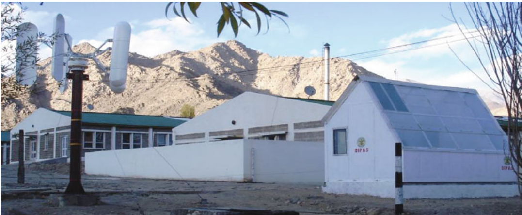
Fig. 2 Solar shelter along with vertical axis wind turbine installed at high altitude (Leh, Ladakh)
