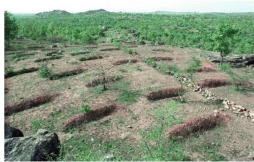
Fig. 8.5 Staggered contour trenching
