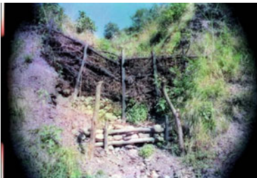
Fig. 8.3 Temporary brushwood check dam
