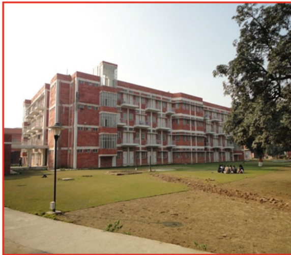
Fig. 1 Data collection site building
