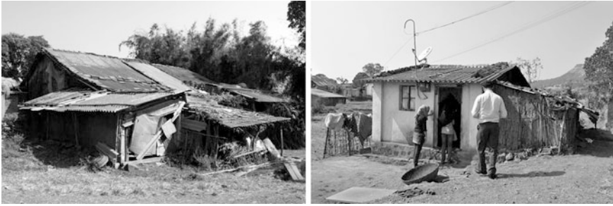
Fig. 1 Self-funded local ( left ) built using local and discarded reusable materials and IAY funded house ( right ) designed and built by a beneficiary himself
