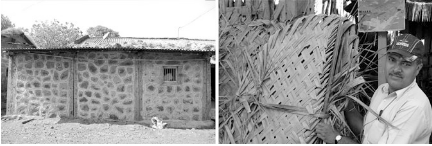
Fig. 3 Precast fencing posts with random rubble in-fills ( left ) and a building material supplier showing palm leaf panels to be used as in-fills in local houses ( right )
