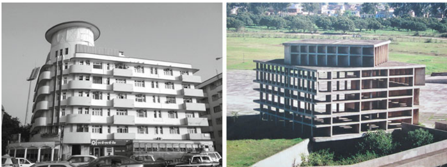
Fig. 4 Modern tropical architecture is very present in India since the 1920s using traditional principles with new materials and in another formal languages; examples are residences in Mumbai and the buildings in Chandigarh
