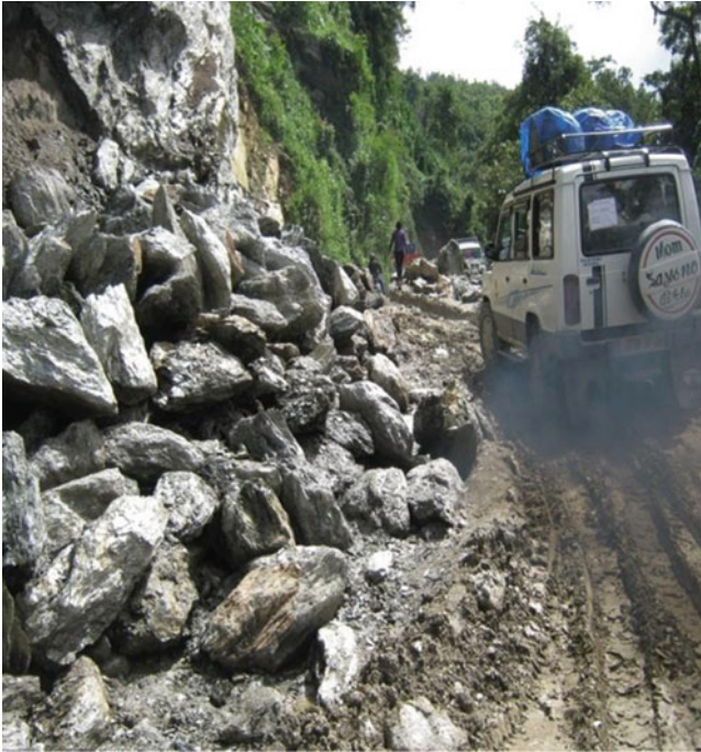
Fig. 4-1 Road clearance made up to Mangan, North Dist. HQ., in 3 days time after the earthquake, but long-term performance measures not ensured, thus affecting work of power projects
