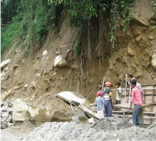
Fig. 4-2 Road widening along NH31A near Ranipool is on but technical feasibility of taming cut slope as seen here are very much local and pristine
