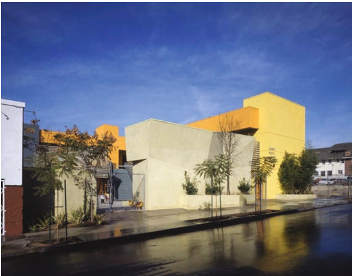
Fig. 12-4. A converted retail shopping center, or mini-mall, by Daly, Genik Architects is now an academically challenging school for the surrounding Central American residents. Photo Credit: Tom Bonner
