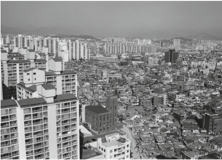
Fig. 3-4. Example of inner city renewal: residential redevelopment sites are shown with the existing low-rise area
