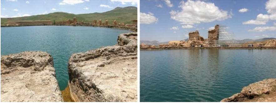
Fig. 5.3 Views of an outlet and vestiges around Takht-e Soleyman-site lake and the remains of Khosrow’s Iwan (right)
