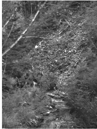
Fig. 2. Large-scale landslide in which bedrock was broken
