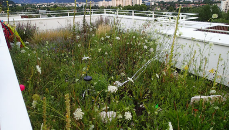
Fig. 3.41 Planted semi-extensive roof garden and then 2 years later (Photo Mr Billic)
