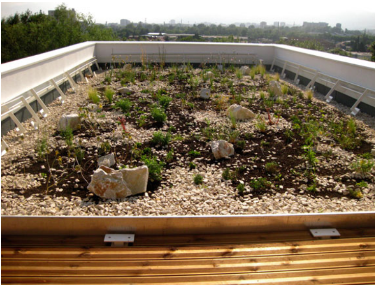
Fig. 3.40 Planted semi-extensive roof garden
