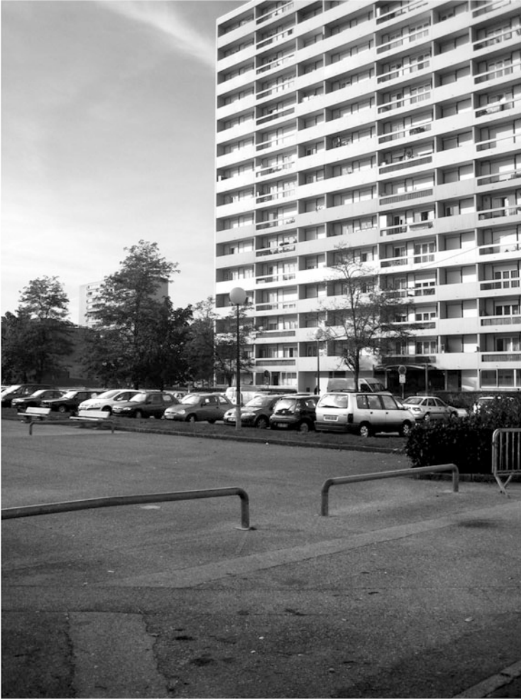
Fig. 3.14 The site before 2008
