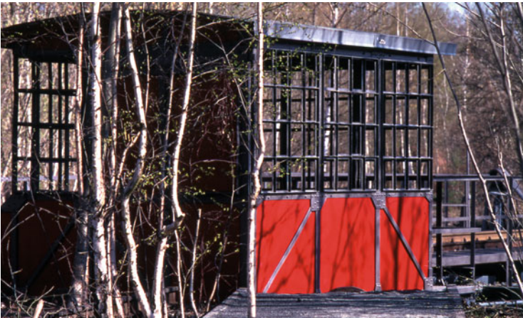
Fig. 2.16 The old turntable was restored (Photo: A. Langer)
