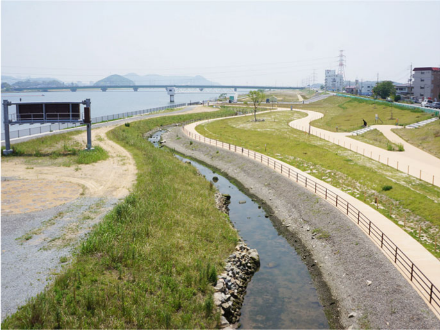
Fig. 5.7 Completed river bank and fishway (2013)
