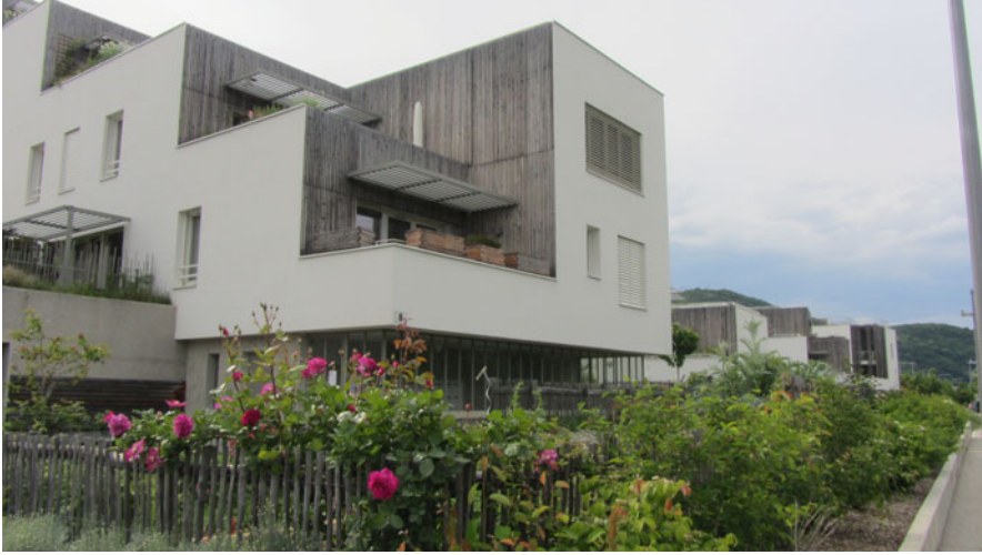
Fig. 3.37 View from south east
