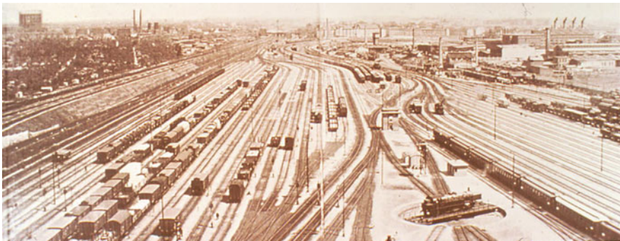
Fig. 2.1 View of the rail-yard in the 1930s (Photo: C. Bellingrodt)
