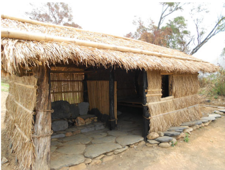
Fig. 7.15 A work hut
