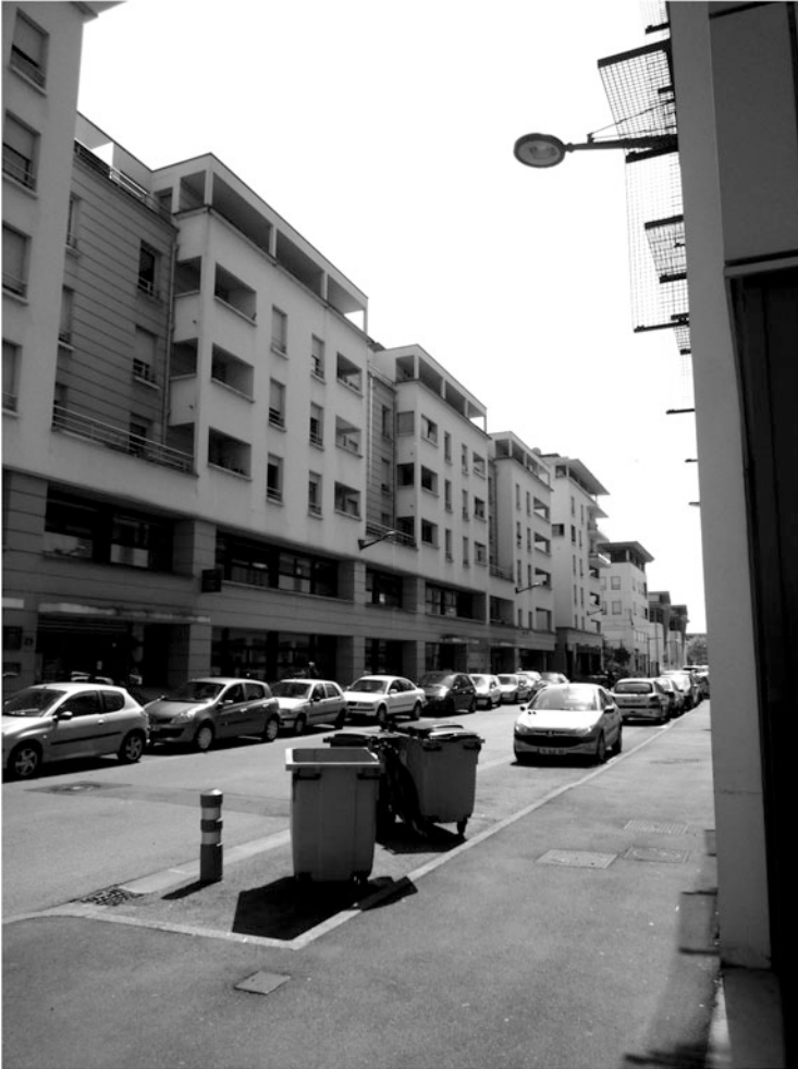
Fig. 3.25 The site before 2010
