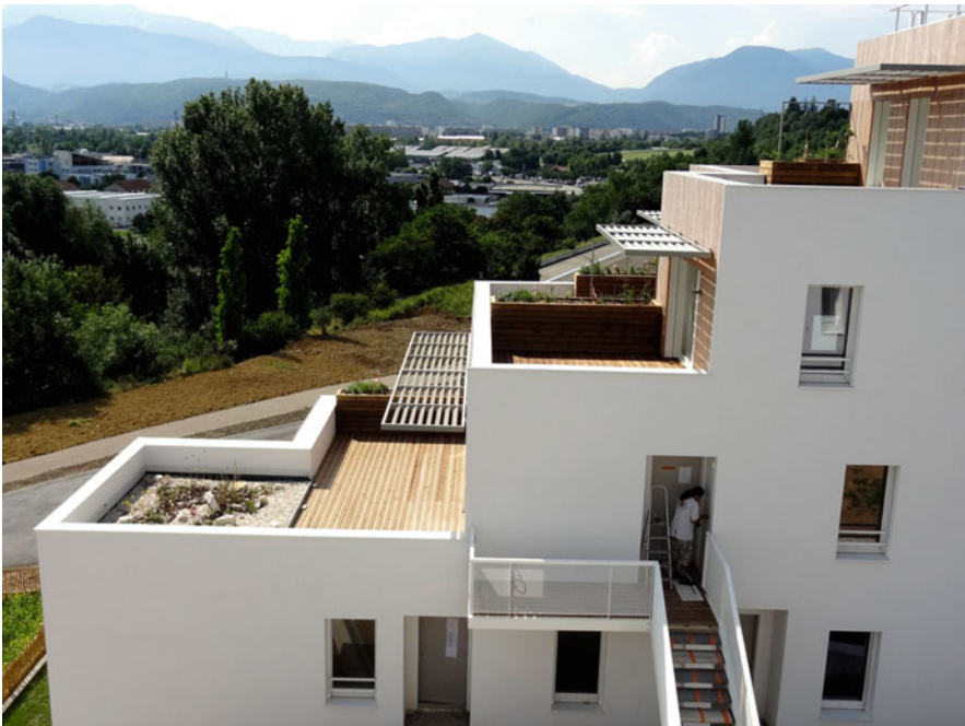
Fig. 3.36 View on terraces
