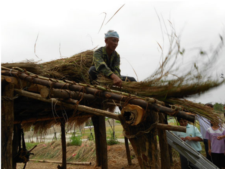
Fig. 7.14 A tribe teacher demonstrated laying out thatched roof
