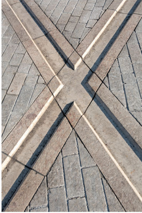
Fig. 3.6 The stone water collectors or gutter system— Albert Videt photo credits
