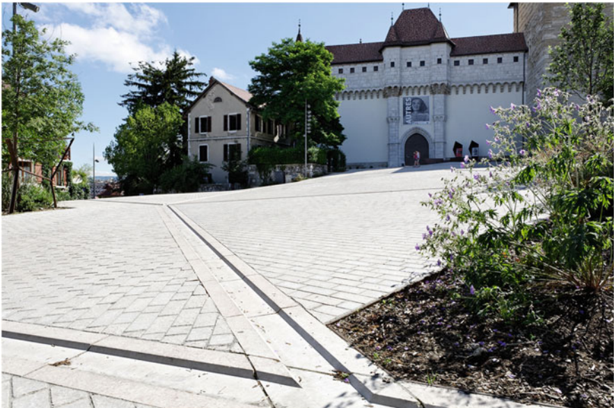
Fig. 3.7 The stone gutters
