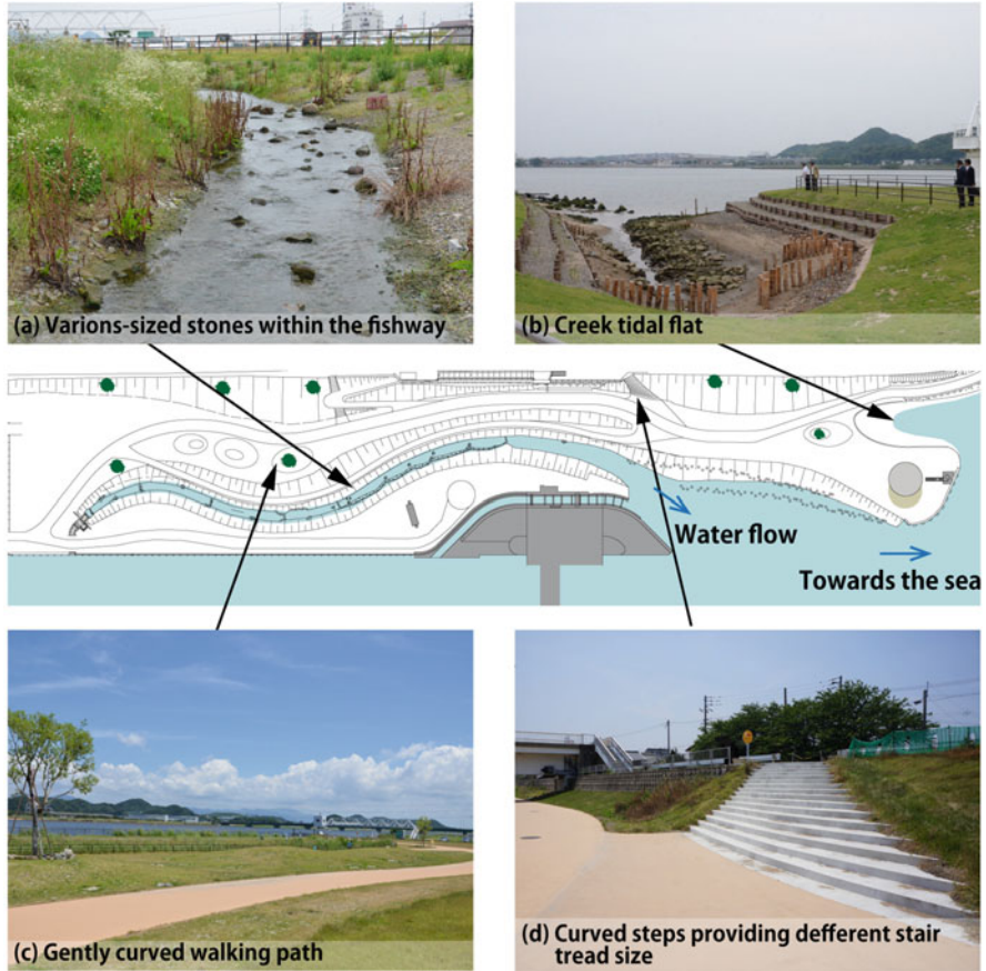
Fig. 5.8 Designed environment of river bank fishway and surroundings. (a) Various-sized stones within the fishway. (b) Creek tidal flat. (c) Gently curved walking path. (d) Curved steps providing different stair tread size
