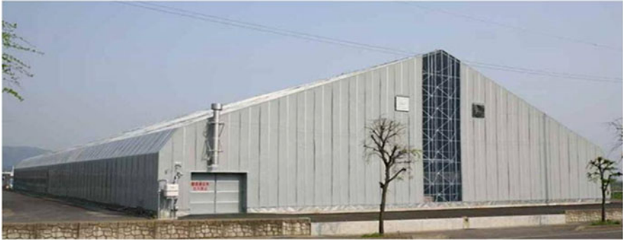
Fig. 7.10 Exterior view of the commercial ISPS plant in Myoko City, Niigata Prefecture
