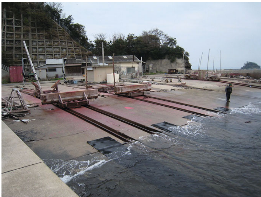
Fig. 2.4 Example of repainting facilities in a fishing harbor. There are three sets of carts and rails to haul boats up a concrete slope. The red paint color adheres to the slope and carts
