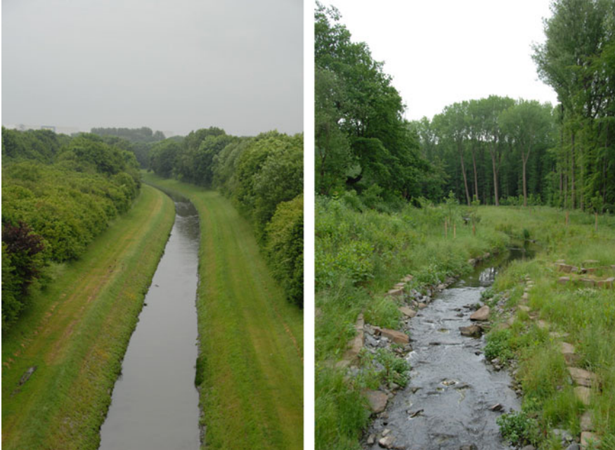
Figs. 18.3 and 18.4 Comparison of two Emscher sections: the Emscher canal in Dortmund-Mengede ( left ) and the revitalized Emscher river in Dortmund-Barop ( right )
