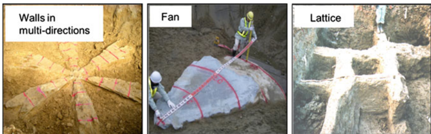
Fig. 10 Views of excavated stabilized soil column in in situ performance verification tests
