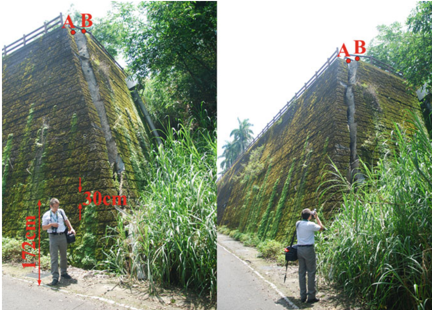
Fig. 5 Image pair for solving relative orientation of the retaining wall failure case
