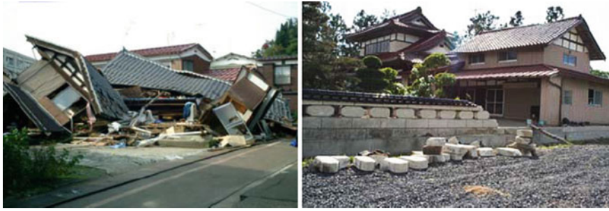
Fig. 1 Comparison of the lightly damaged house, which was built in 1980, Iwate–Miyagi inland earthquake, 2008 ( M_j 7.2), Ishinomaki, Miyagi prefecture ( left photo taken in 15 June, 2008) and the collapsed house in Niigata Chuetsu-Oki earthquake, 2004 ( M_j 6.8), Kawaguchi, Nigata, prefecture, ( right photo taken in Oct., 2004)
