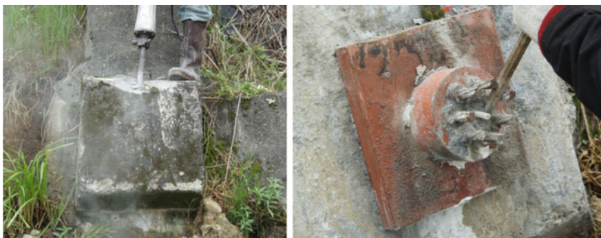
Fig. 7 Remove the concrete protection cap of anchor head
