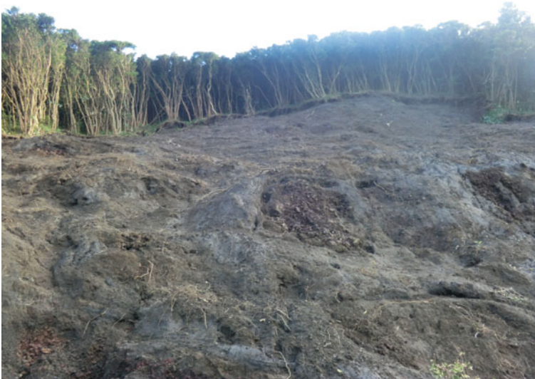
Fig. 16 Actual slope surface observed after disaster
