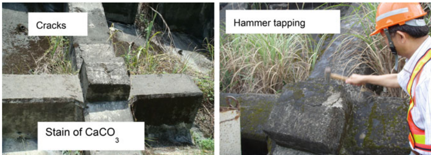
Fig. 6 Visual inspection and hammer tapping on the concrete cap of anchor
