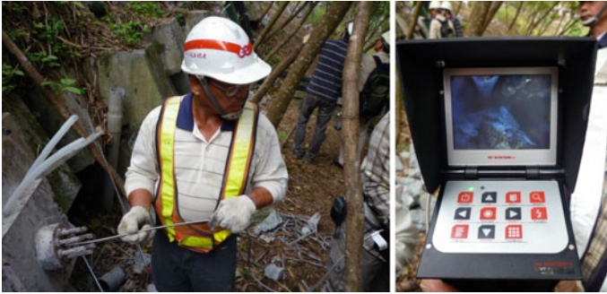
Fig. 8 Use endoscope to inspect steel strands under the anchor head
