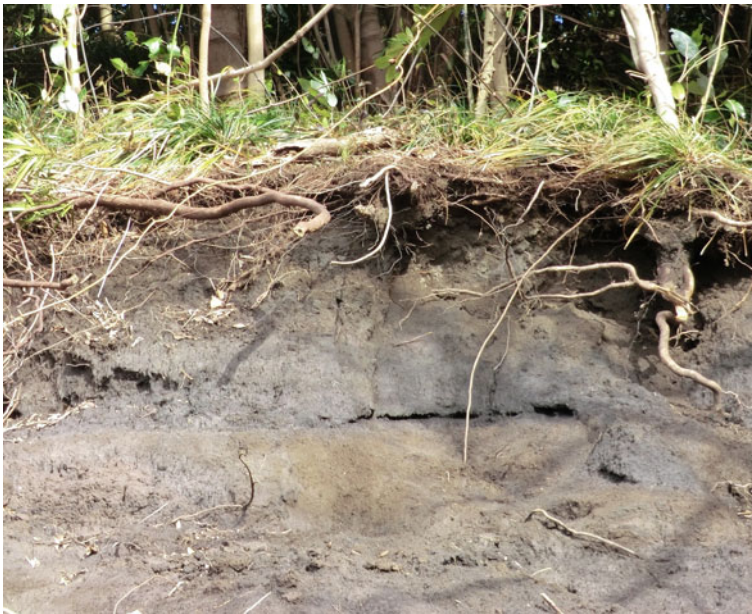
Fig. 2 Many small holes of local scouring along thin ash-fall deposit layer
