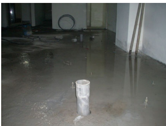
Fig. 6 Pre-embedded outer pipe
