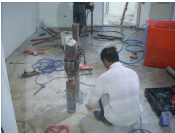
Fig. 5 Drilling hole on the foundation slab
