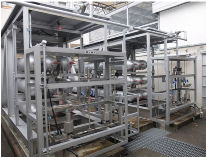
Fig. 2.12 Hydrogen tanks for high-pressure hydrogen storage (inside the hydrogen filling station at Kyushu University)
