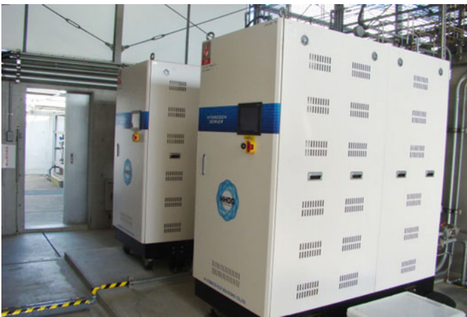
Fig. 2.11 Polymer electrolyte fuel cell (PEFC)-type water electrolysis system (inside the hydrogen filling station at Kyushu University)
