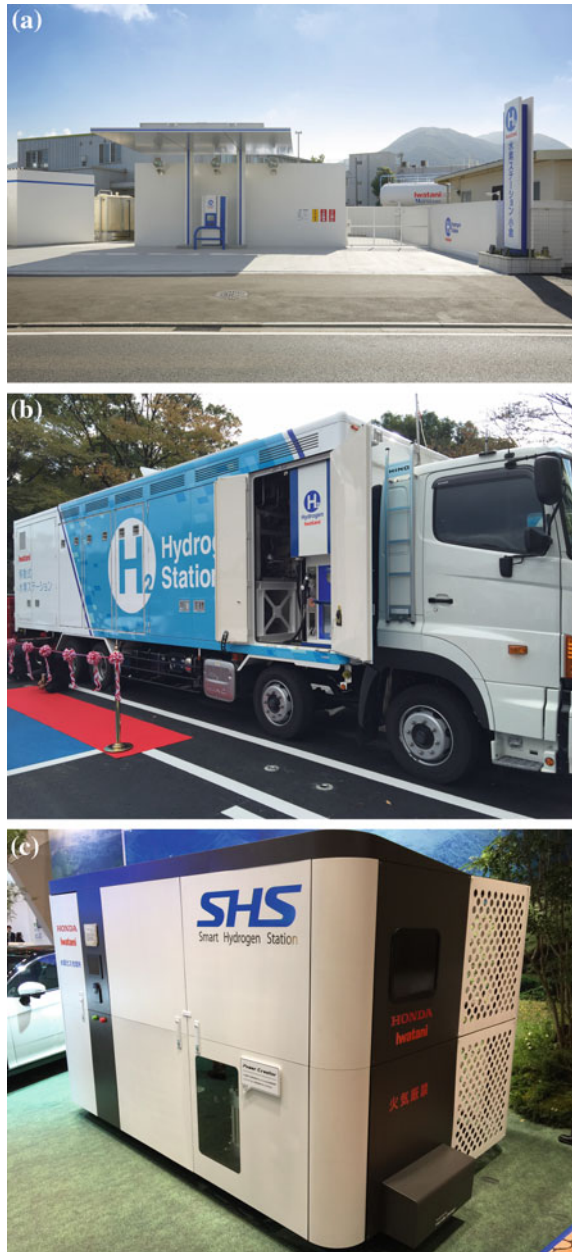
Fig. 2.3 Hydrogen filling stations: a the Kokura hydrogen filling station (stationary, 70 MPa), which was the second such station to open to the general public in Japan, on October 22, 2014; b the Fukuoka Prefecture hydrogen filling station (mobile, 70 MPa); and c a small-scale hydrogen filling station “Smart Hydrogen Station (SHS)” (35 MPa) developed by Honda and Iwatani exhibited in Tokyo Motor Show 2015
