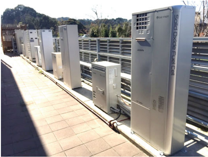
Fig. 2.7 Various types of ENE-FARM fuel cell units for residential use. The ones shown here are installed on Ito Campus at Kyushu University
