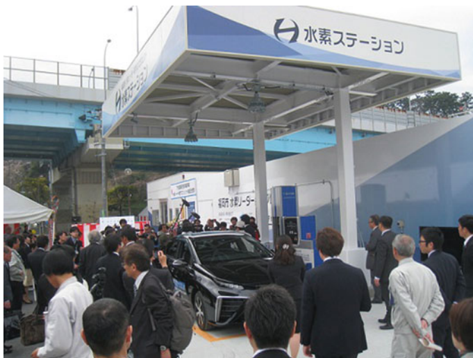
Fig. 1.6 A renewable hydrogen filling station in Fukuoka City, where hydrogen gas is produced from digestion gas consisting of CH 4 and CO 2
