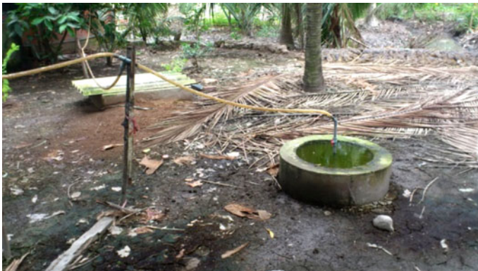
Fig. 8.4 Dome-type biogas digester installation in Vietnam (July 2013)
