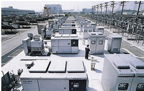
Fig. 5.13 14 units of 50 kW phosphoric acid fuel cells (PAFCs) at Rokko. Source NEDO
