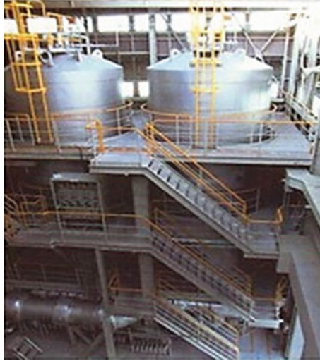
Fig. 5.19 250 kW stack. Source FCDIC
