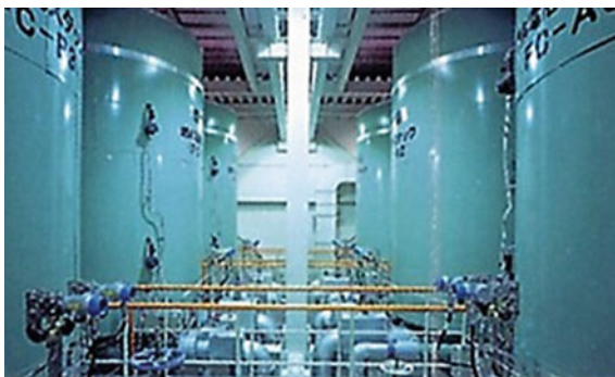
Fig. 5.14 5 MW phosphoric acid fuel cell (PAFC) stacks by Fuji Electric Co. Source Fuji Electric Co.
