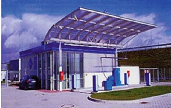
Fig. 4.33 Hydrogen station at Munich airport
