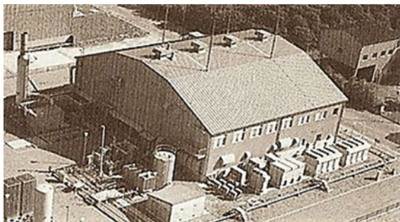
Fig. 5.10 1 MW phosphoric acid fuel cell (PAFC) plant at Kansai Electric Power. Source AIST
