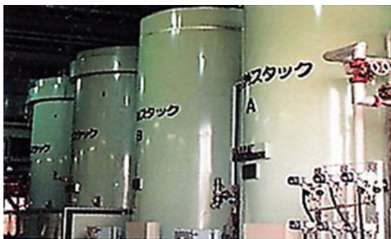
Fig. 5.9 Phosphoric acid fuel cell (PAFC) stack, 250 kW \times 4 units. Source Fuji Electric Co.
