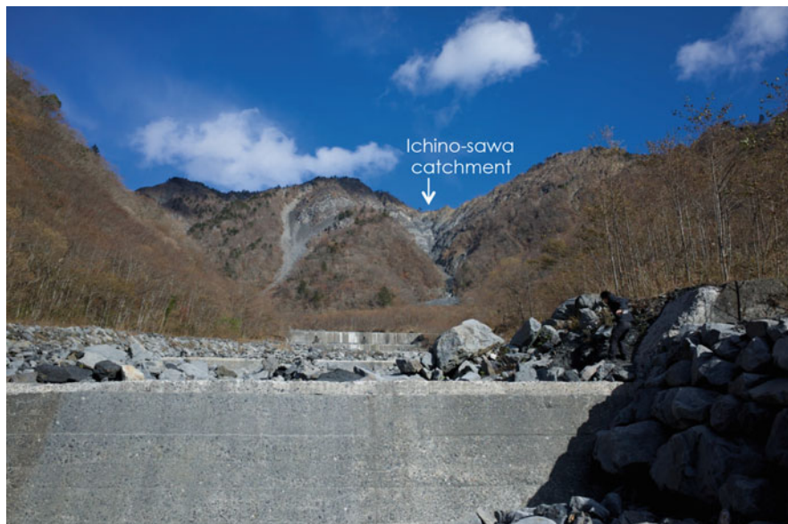
Fig. 8.2 Artificial check dams in the Ohya-kuzure landslide along a tributary of the upper Abe-kawa River. Quite many dams have been constructed for “sabo” erosion control work in this area. The entire photograph shows a part of the area of the Ohya-kuzure landslide terrain, and the study site, the Ichino-sawa catchment, is shown in the central left of the photograph
