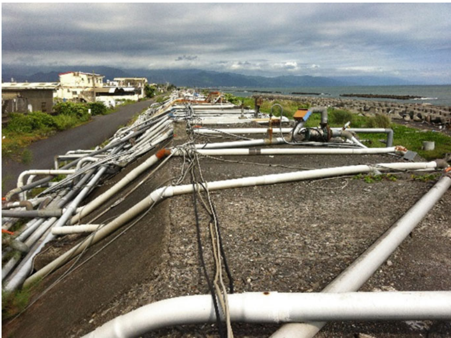
Fig. 7.5 Water pipes conveying seawater into aqua farms (Source: taken by author, Jia-tung Township, Pingtung County, July 2014)
