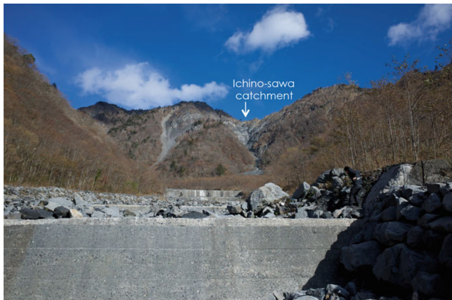
Fig. 8.2 Artificial check dams in the Ohya-kuzure landslide along a tributary of the upper Abe-kawa River. Quite many dams have been constructed for “sabo” erosion control work in this area. The entire photograph shows a part of the area of the Ohya-kuzure landslide terrain, and the study site, the Ichino-sawa catchment, is shown in the central left of the photograph
