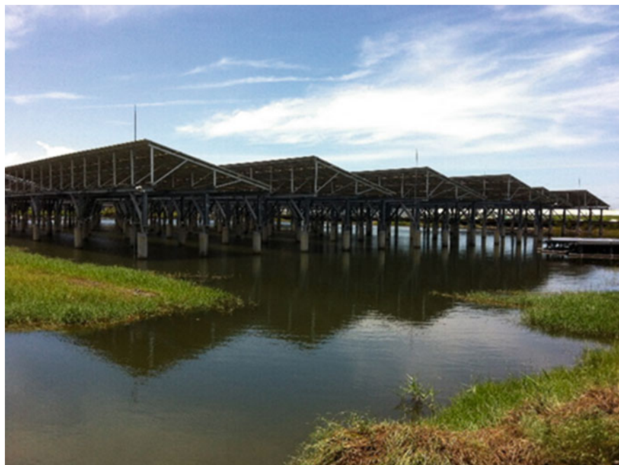
Fig. 7.7 A view of the solar energy farming plant in Jia-tung township (Source: taken by the author July 2014)
