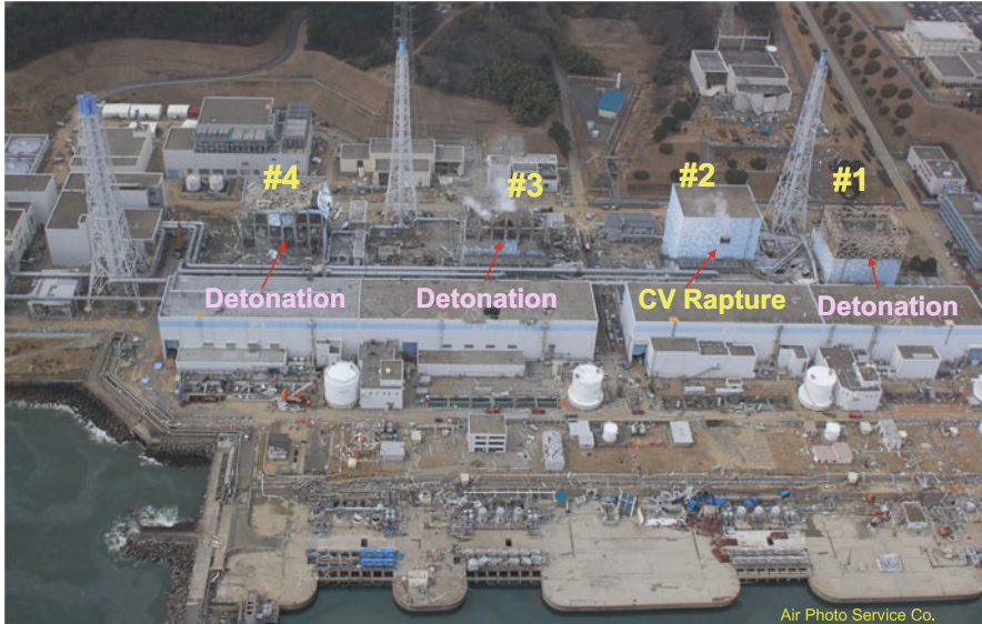
Fig. 8 H 2 detonations occurred after vent operations (Units 1, 3, and 4) [11]
