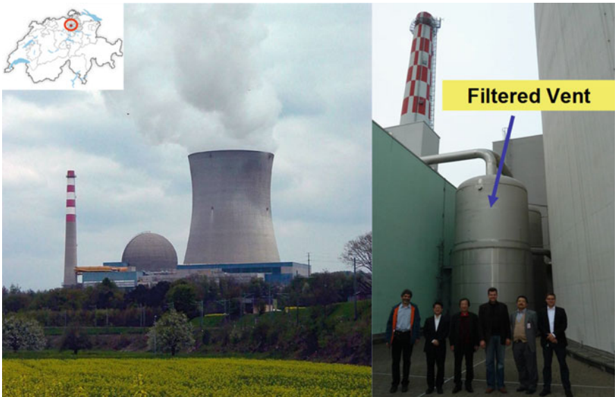
Fig. 20 FCVS in Leibstadt NPP (BWR), Switzerland [8]
